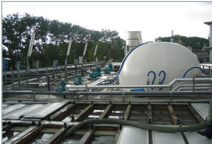
Anaerobic biological treatment tank (credit: Austep SRL)
